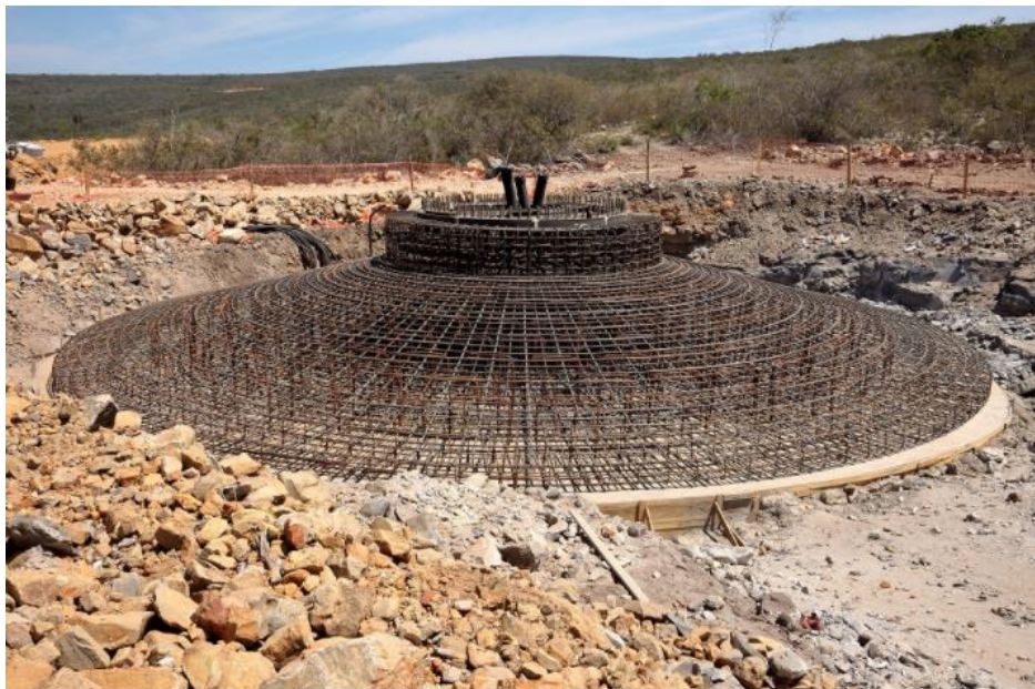
Wind Turbine Foundation
