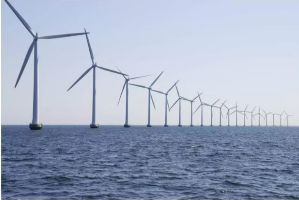
Offshore Wind Energy
