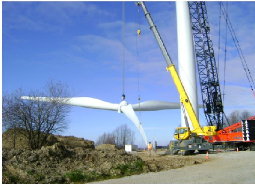
Rotor (blade + hub) being lifted for installation
